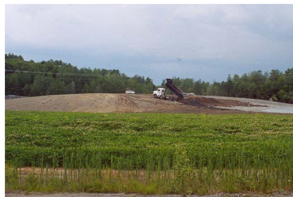
A layer of earth is placed over the low permeability membrane
